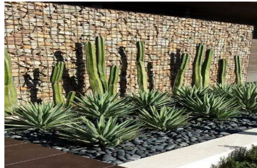
The above is an illustration of a gabion type wall, but the height should be a maximum of 1200 mm.
